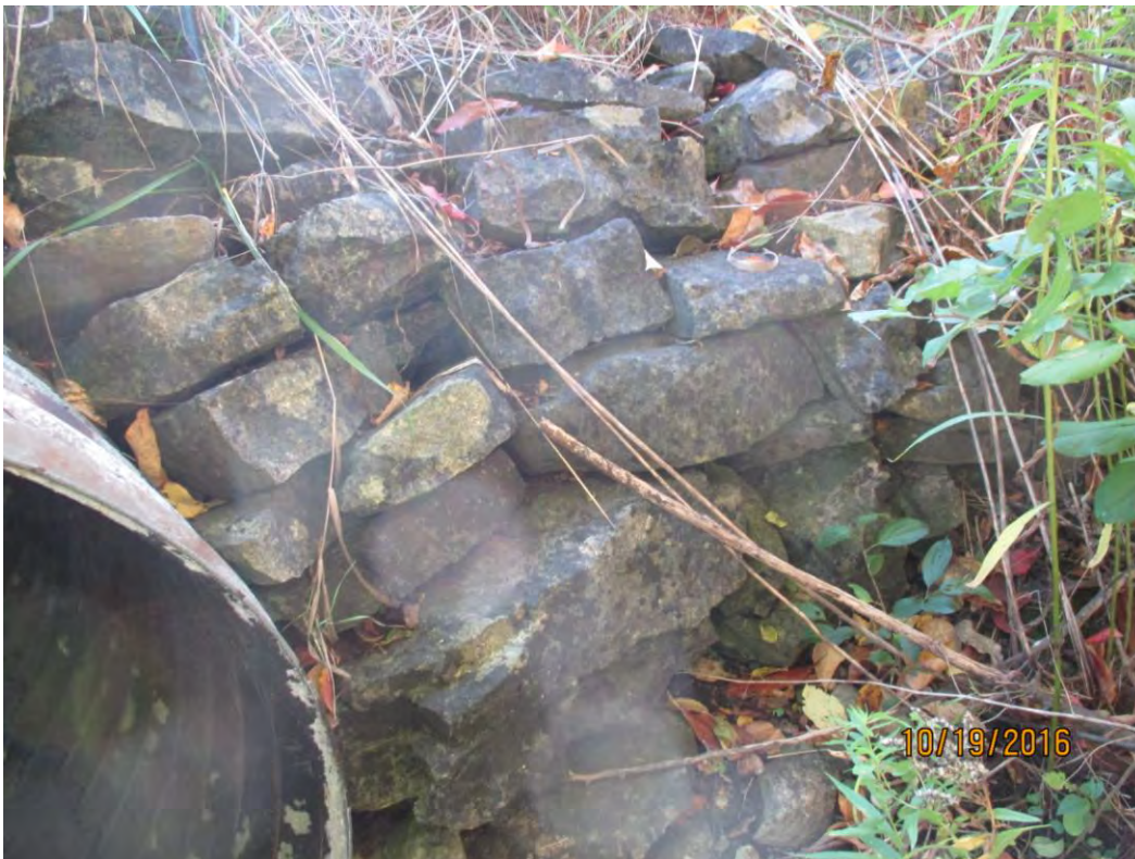
Photo 8: Signs of instability at west retaining wall
