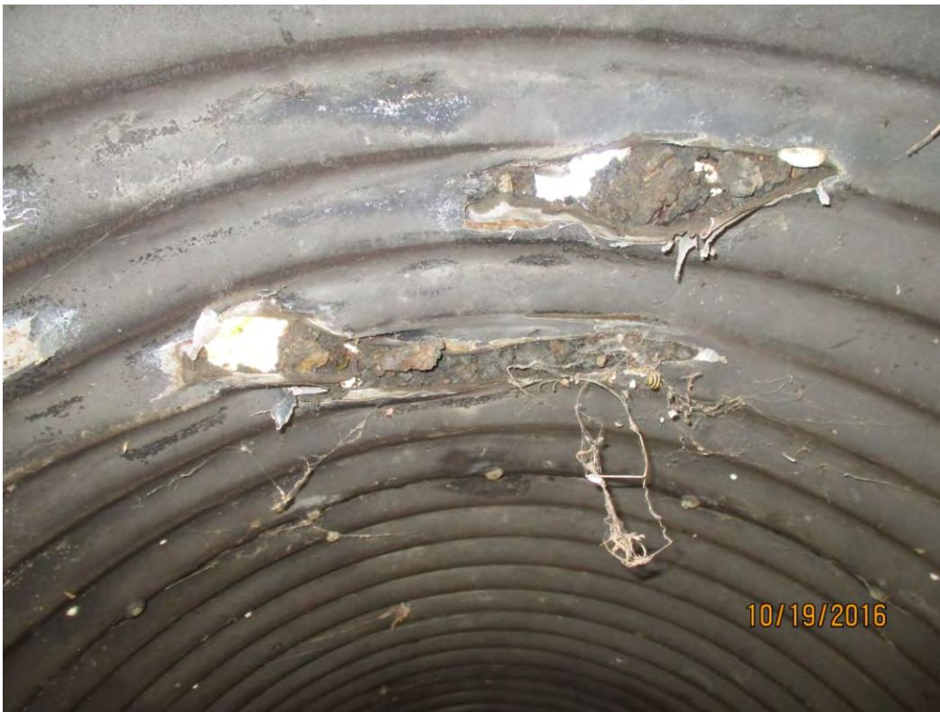
Photo 6: Perforations at top of barrel
