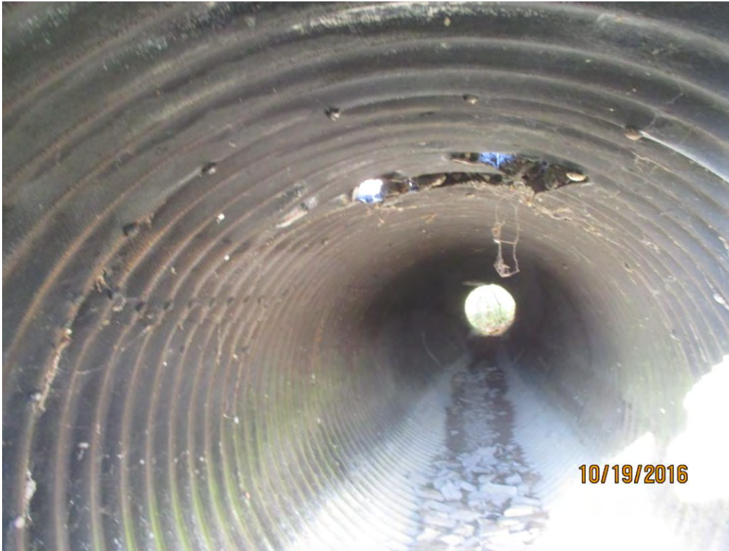
Photo 5: Crushing of barrel
