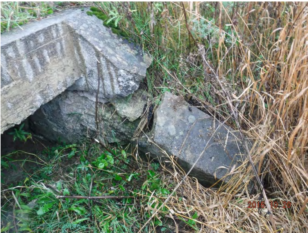
Photo 10: Separation of southwest wingwall
