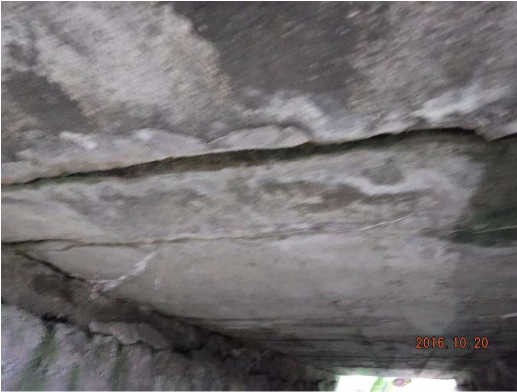
Photo 7: Very wide crack at soffit interior
