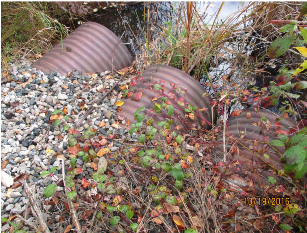
Photo 6: Light corrosion at exposed barrel ends
