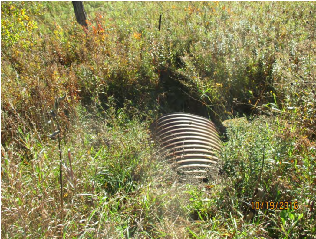
Photo 7: Light corrosion on exposed barrel exterior
