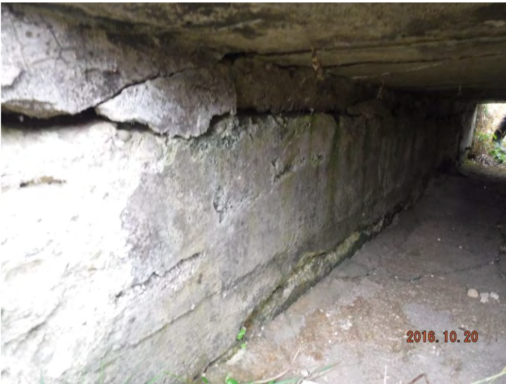
Photo 8: Severe deterioration of north abutment wall
