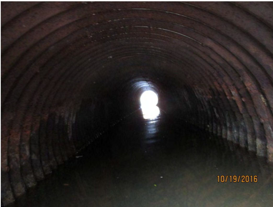
Photo 4: Medium to severe corrosion at barrel interior
