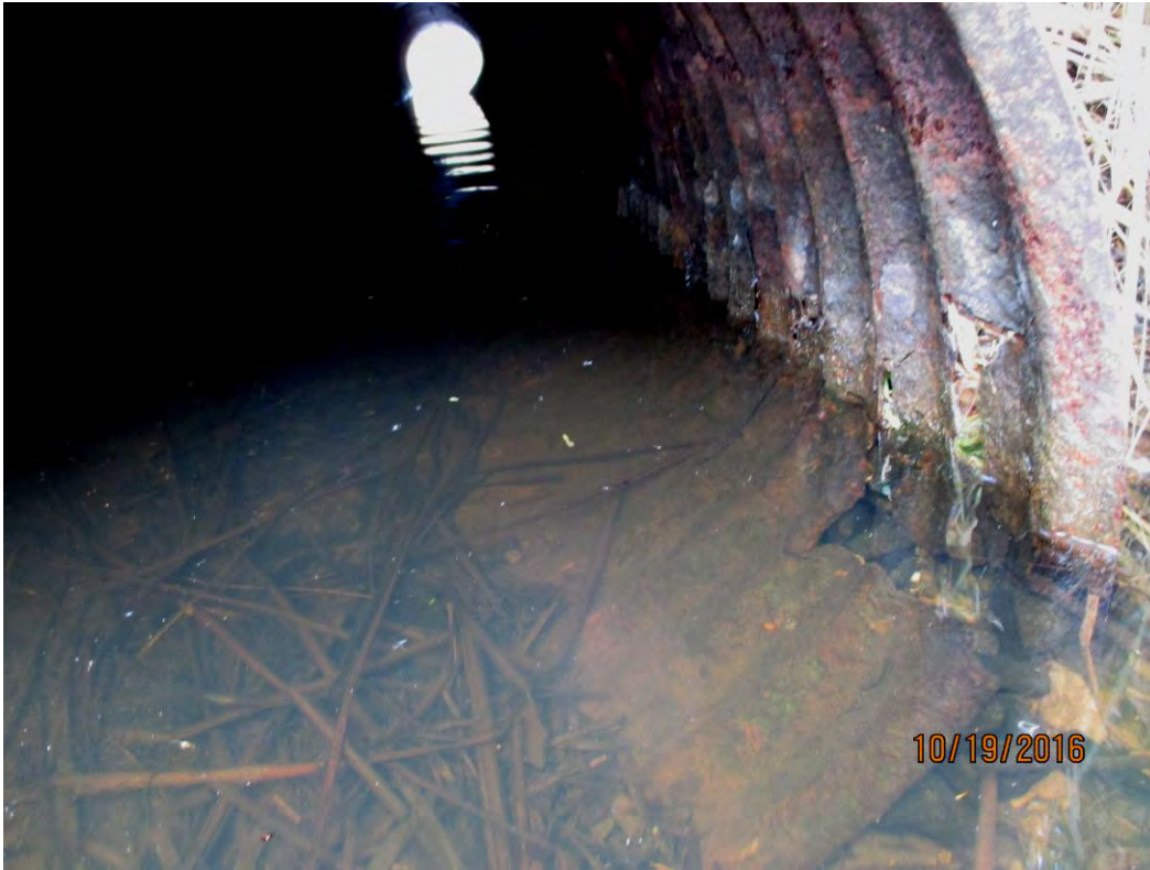
Photo 5: Severe corrosion and perforations at west end of north barrel
