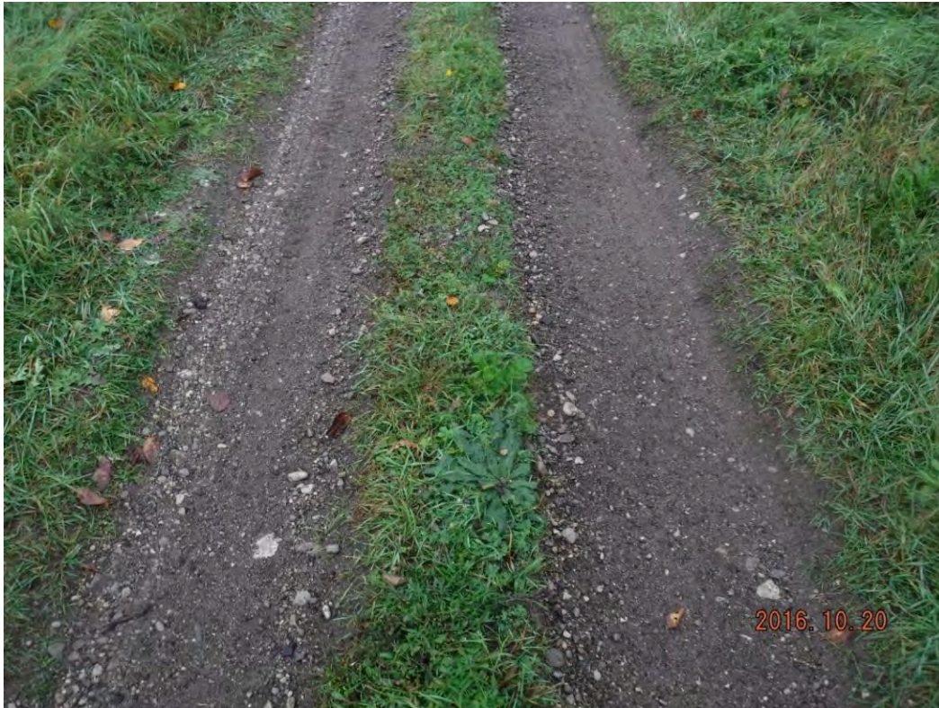
Photo 5: Medium to severe wheel track rutting and vegetation on approaches
