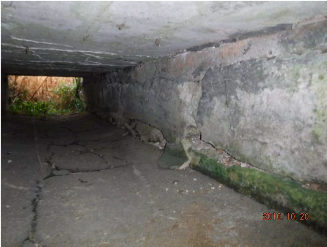
Photo 9: Severe deterioration of south abutment wall
