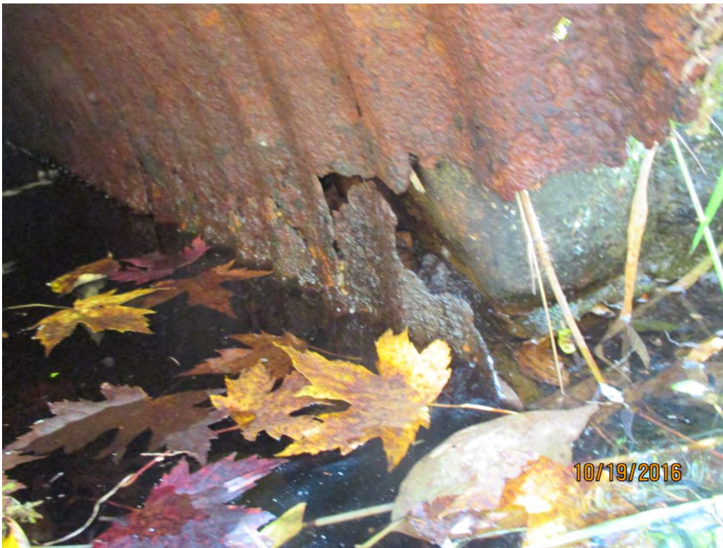
Photo 6: Severe corrosion and perforations at west end of barrel
