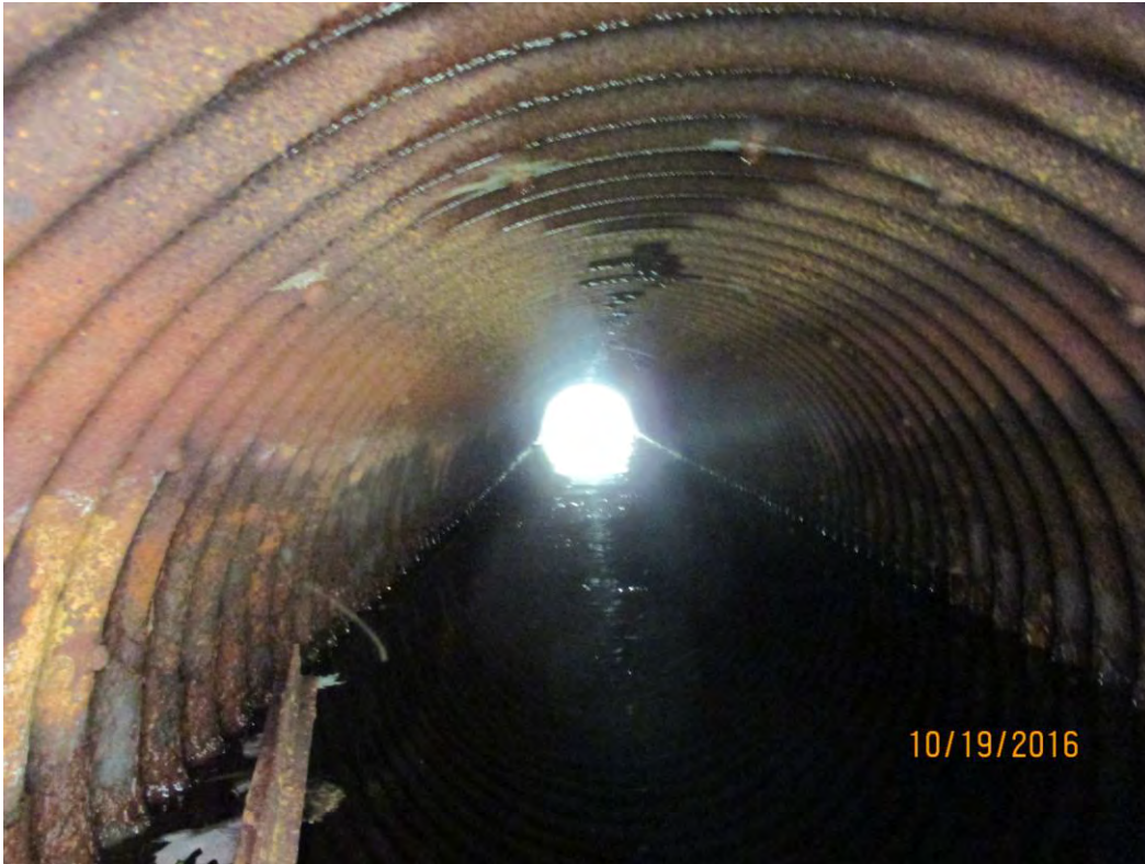
Photo 5: Medium to severe corrosion at barrel interior
