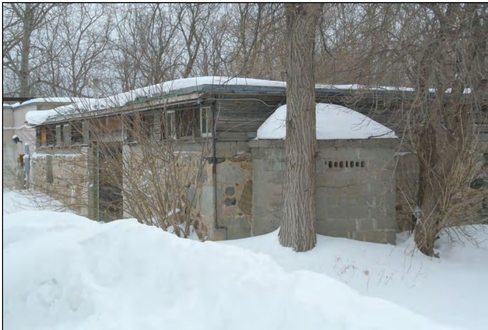
Plate 4: Detail of the southwest and southeast elevations. Note the concrete block addition.
