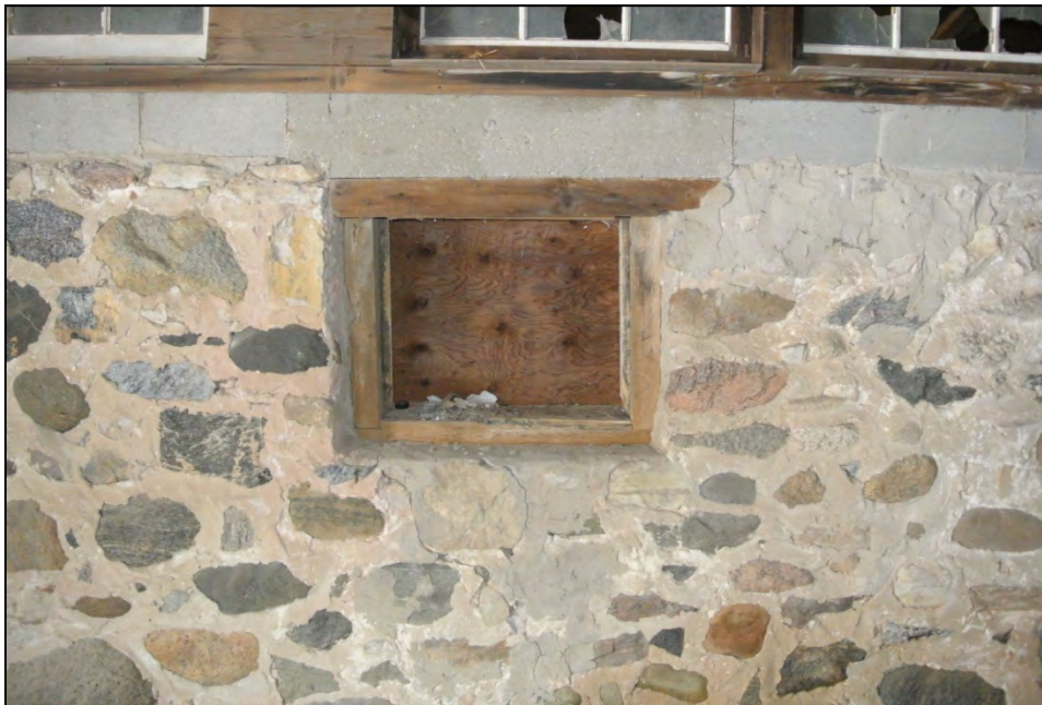
Plate 18: Window in northeast stone wall of the original structure. Note the wood frame and line of concrete blocks directly above.
