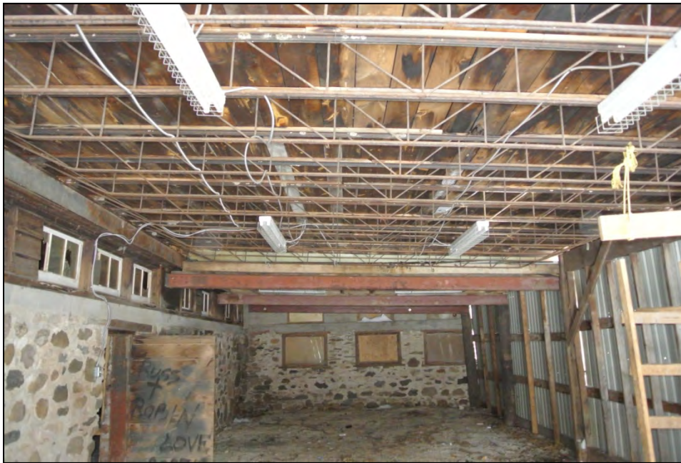
Plate 25: Detail of wood-slat and truss ceiling.
