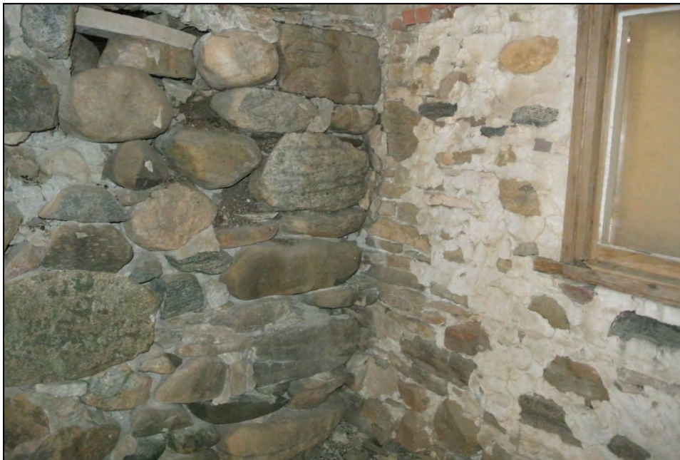
Plate 26: Detail of northwest corner of driveshed. Note the different stonework used to complete the original structure (left) and the contemporary addition (right).
