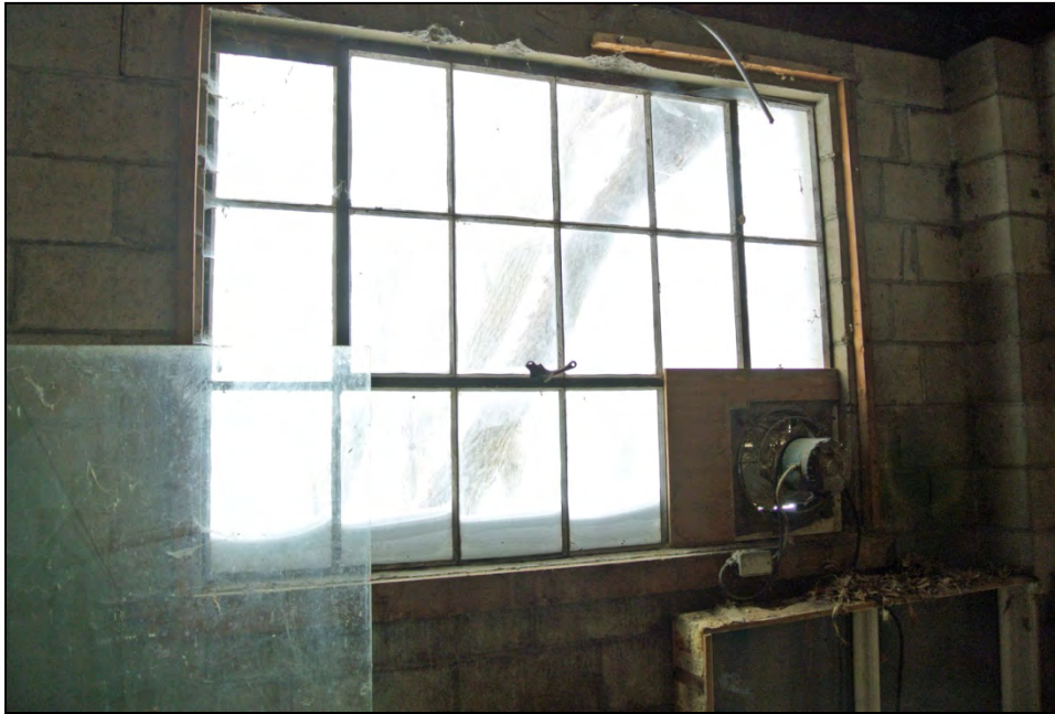
Plate 23: Detail of 18 pane window with metal muntins and eight-pane, central outward-opening panel.
