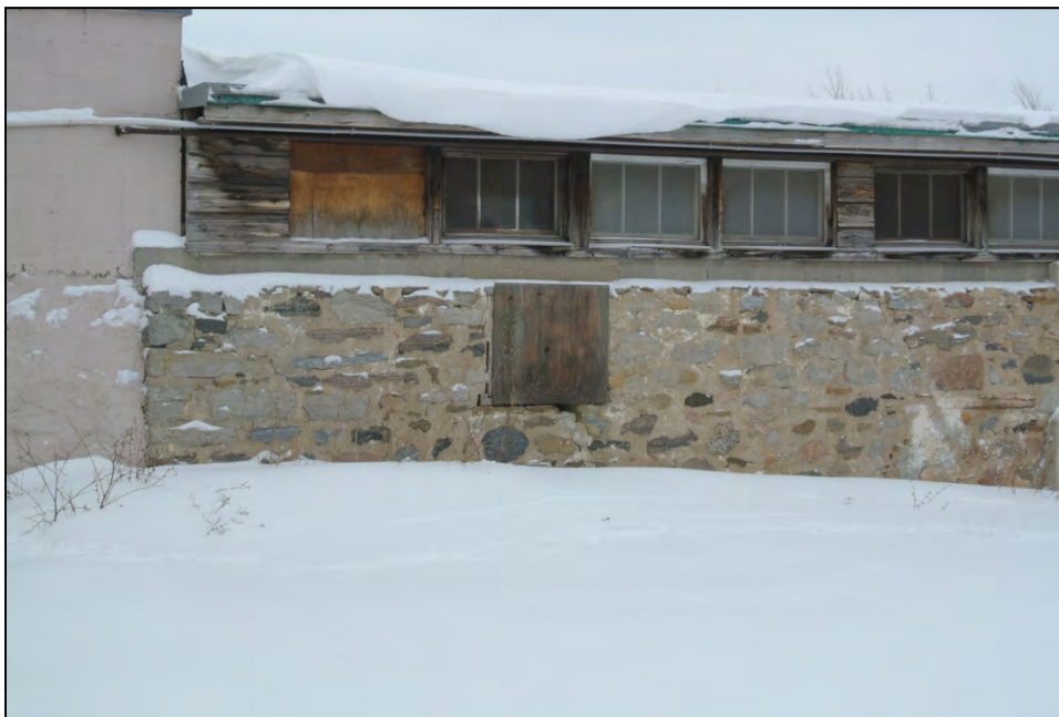
Plate 14: Detail of southwest wall of original structure. Note the wood frame resting atop a row of concrete blocks above the stone wall.
