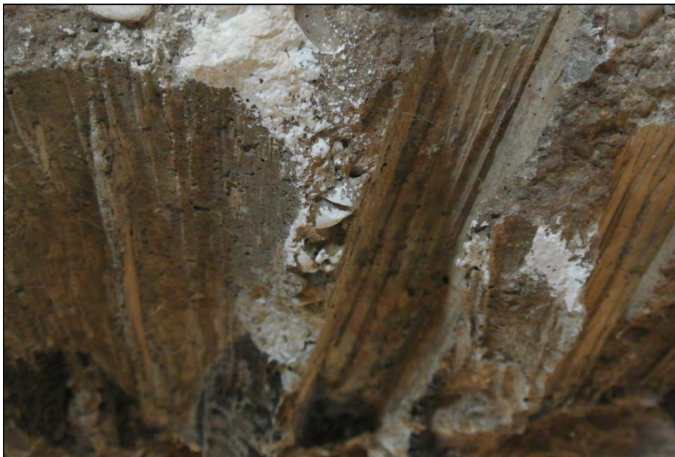
Plate 46: Detail of door opening into modern addition two. Note the distinctive marks in the concrete above the doorway left by the cordwood wall.
