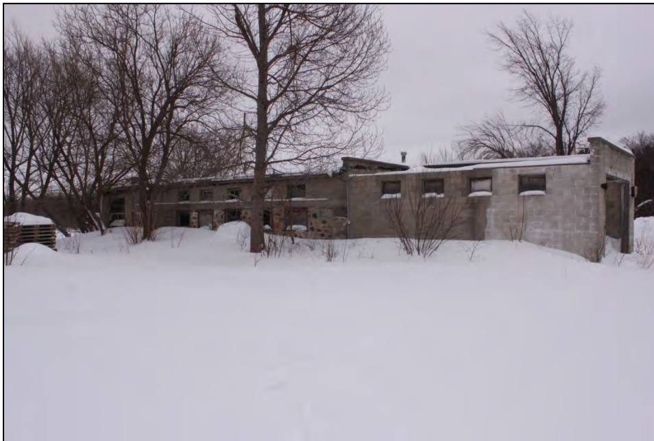
Plate 6: Northwest elevation of building. Note the concrete block garage, the large stone addition, and the small addition on the northeast side of the building.
