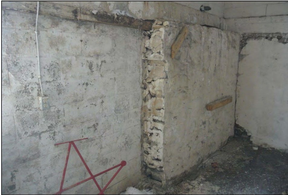
Plate 43: Detail of northwest wall of historic addition. Note the absence of stone wall revealing the concrete blocks added to the exterior.
