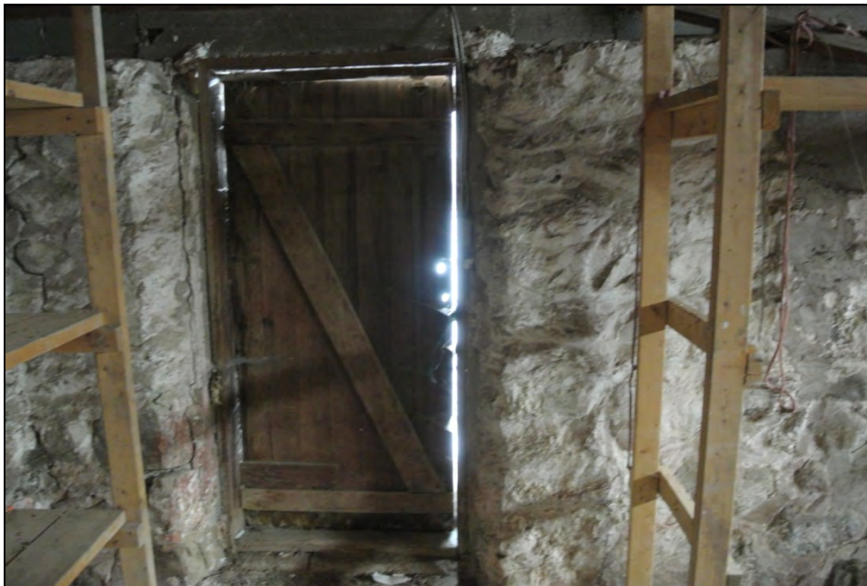
Plate 30: Detail of vertical wood-plank door on southeast elevation of original structure.
