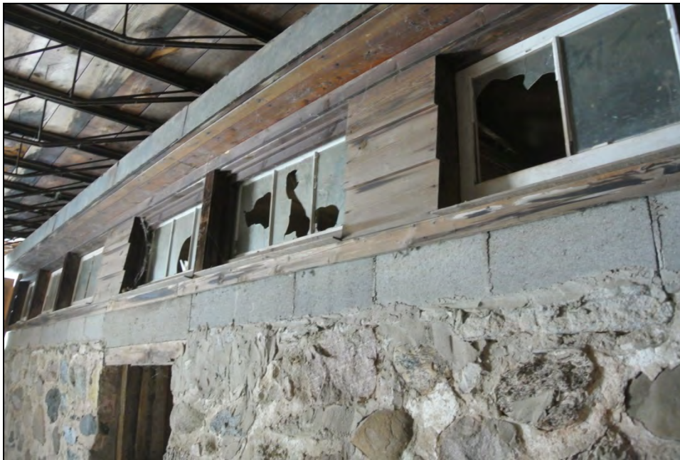
Plate 21: Row of windows in the frame structure above the stone wall.
