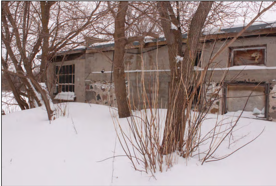
Plate 7: Detail of the northwest elevation. Note the concrete blocks placed upon stone foundations.
