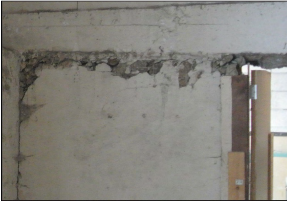
Plate 45: Detail of northwest wall of historic addition. Note that the wall is comprised of plaster and cordwood construction.
