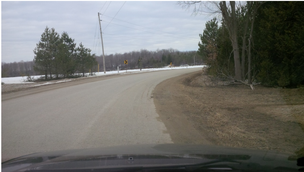
Figure 3: Looking North on North-East Bend of Sideroad 60
