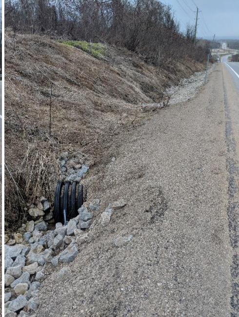
Photo 2 – SC A Culvert Inlet & Roadside Ditch
