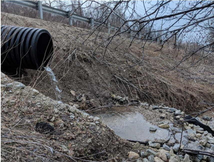
Photo 3 – SC A Culvert Outlet, Slope Erosion, & Coarse Substrate
