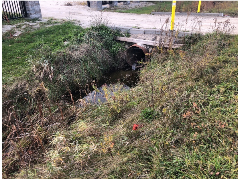
Photo 3: Facing west, the outlet of a driveway culvert with scour pool present. Fish were observed in this location (11-5-2020).
