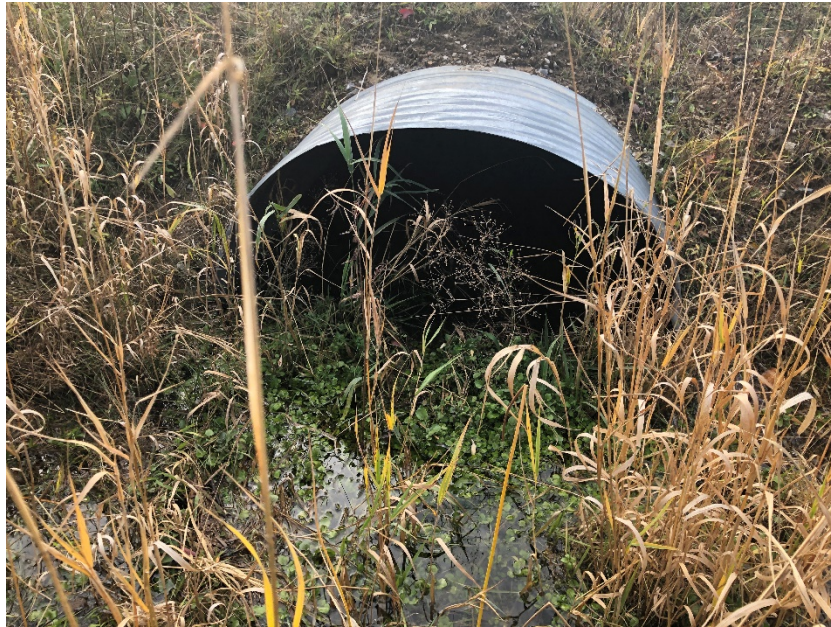
Photo 4: Facing south, the outlet of the CSP beneath GR19 (11-5-2020).
